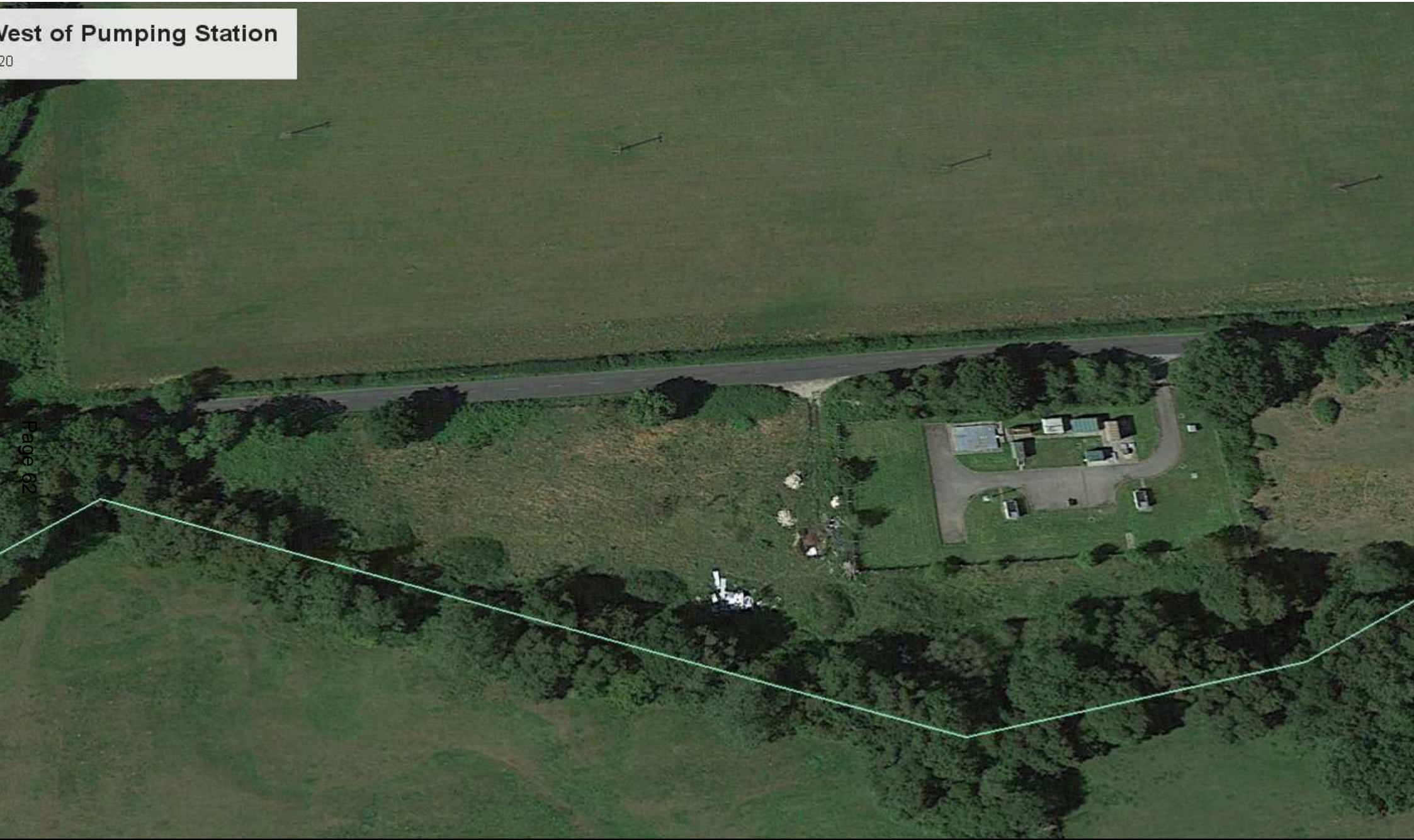
view of application site (Google Earth)
