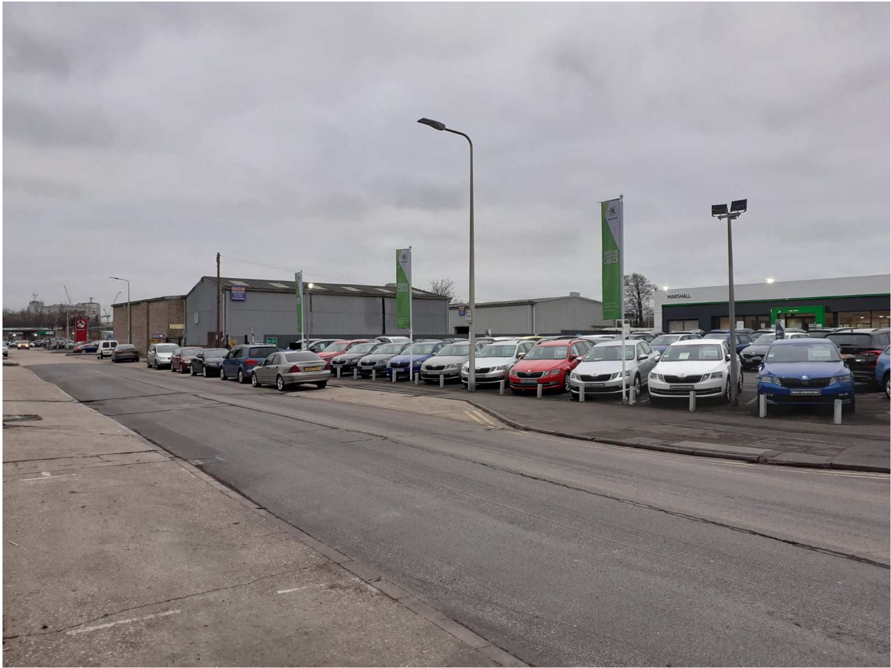
View of application site along Faraday Road (looking South)
